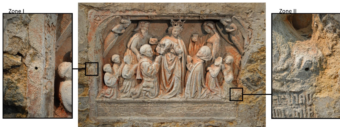
Figure 2: The location of the samples before desalination (left: zone I and right: zone II). Samples after desalination are taken just above the initial samples (not shown). The (testo) probe that was placed in the drill hole shown left (zone I) logged the RH en T during the drying process.
