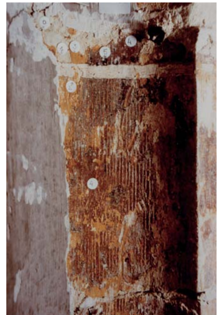
II.4 Examination window showing applied brocade © Lode De Clercq
