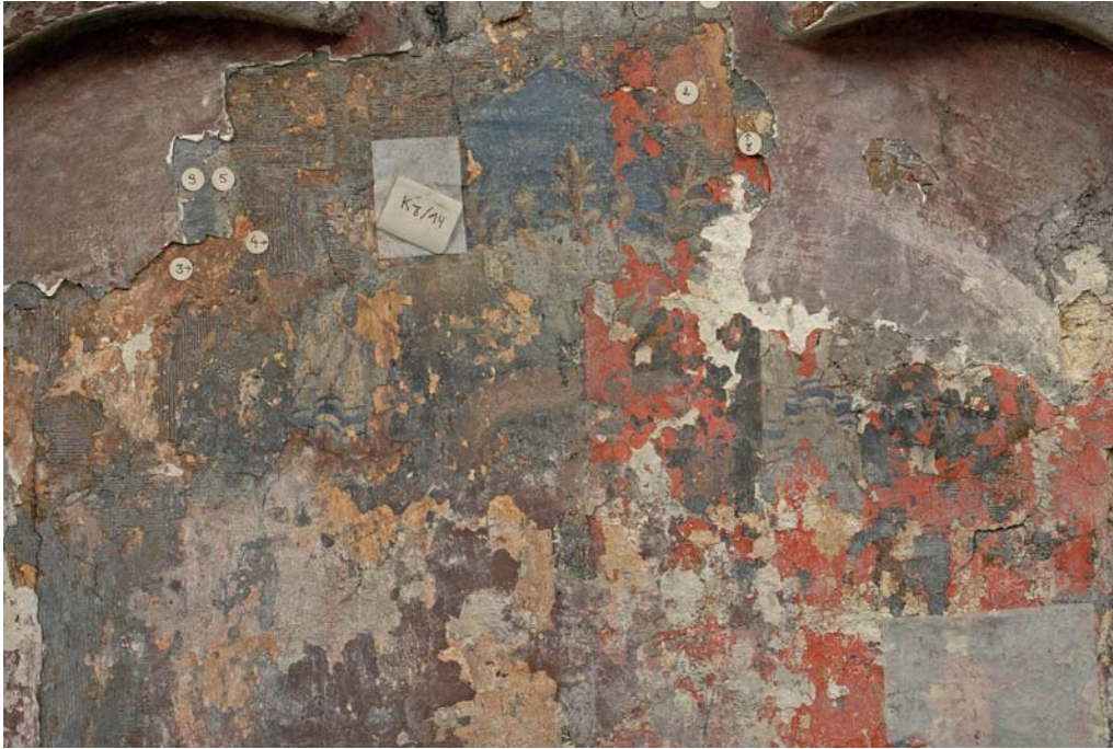
10.1a Right-hand blind arcade with painted figure and applied brocade
