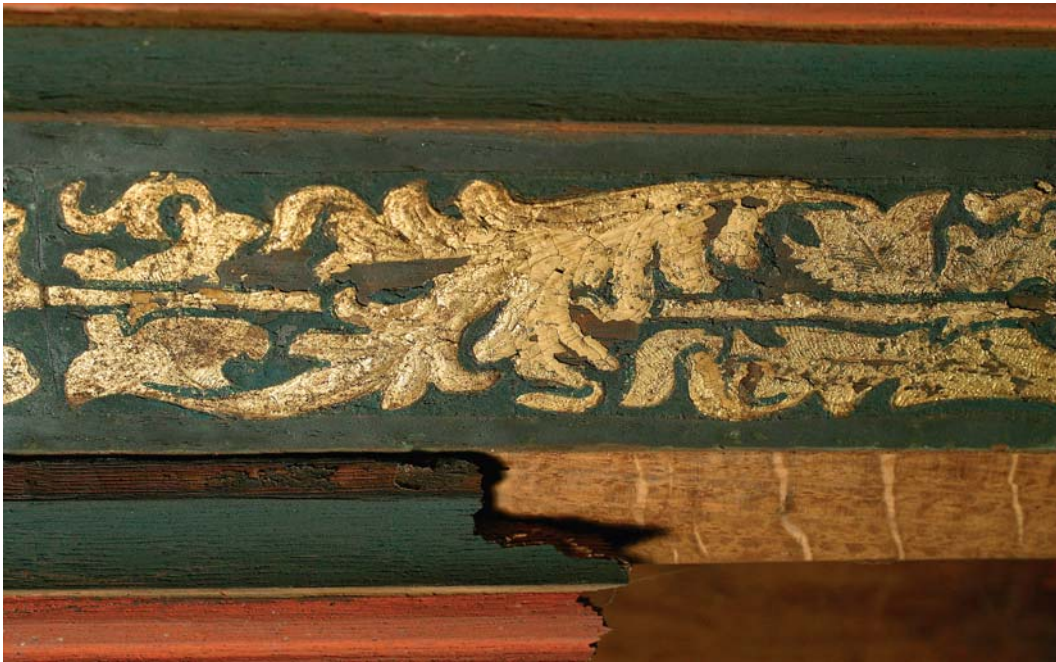
17.1a Applied brocade on the joists of the council chamber ceiling
