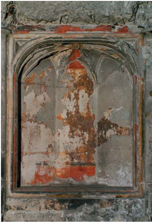
33.1a Applied brocade in the niche
