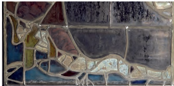
Fig. I.59. Example of extensive corrosion: nIII 3b.
