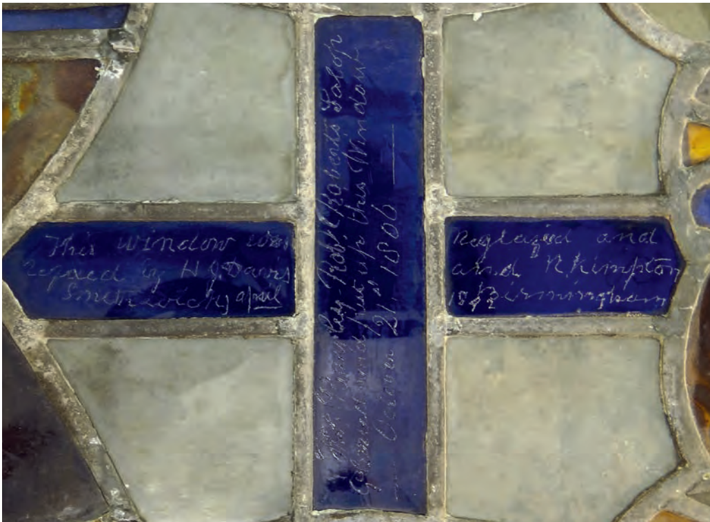
Fig. I.71. Signatures of the late nineteenth-century glaziers H. J. Davis and R. Kimpton (1892) added to those of the early nineteenth-century glaziers Thomas Bayley and Robert Roberts (1806) on the same cross.
