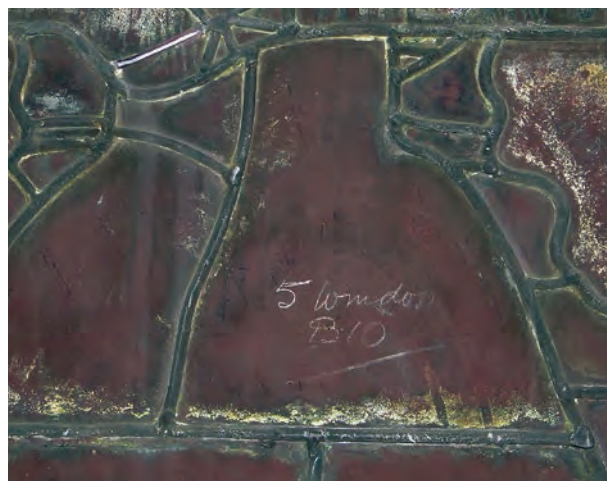
Fig. I.66. Inscription in pencil indicating the position of a panel in a window, specifying the light and the row ('5 window | B10'), 1939 or 1945.
