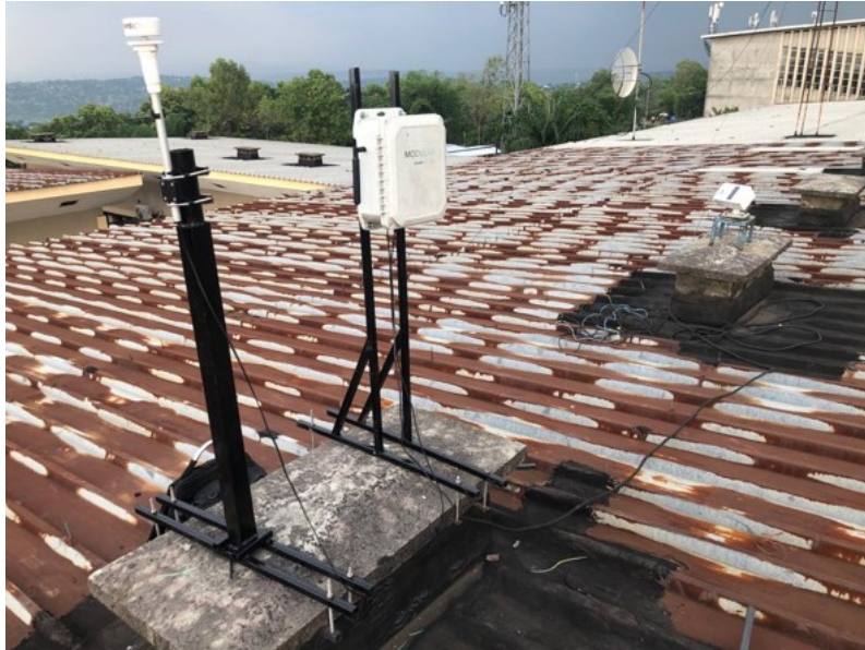
Figure 2.13: Current atmospheric pollutant measurement station located on the rooftop of the Faculty of Sciences at the University of Kinshasa. On the left, the MODULAIR instrument for surface measurements, installed in May 2023, and on the right, the MAX-DOAS instrument, the foundation of this thesis, installed since November 2019. The MAX-DOAS instrument enables measurements at various elevation angles, facilitating the extraction of vertical profiles of trace gases in the UV-Vis range.
