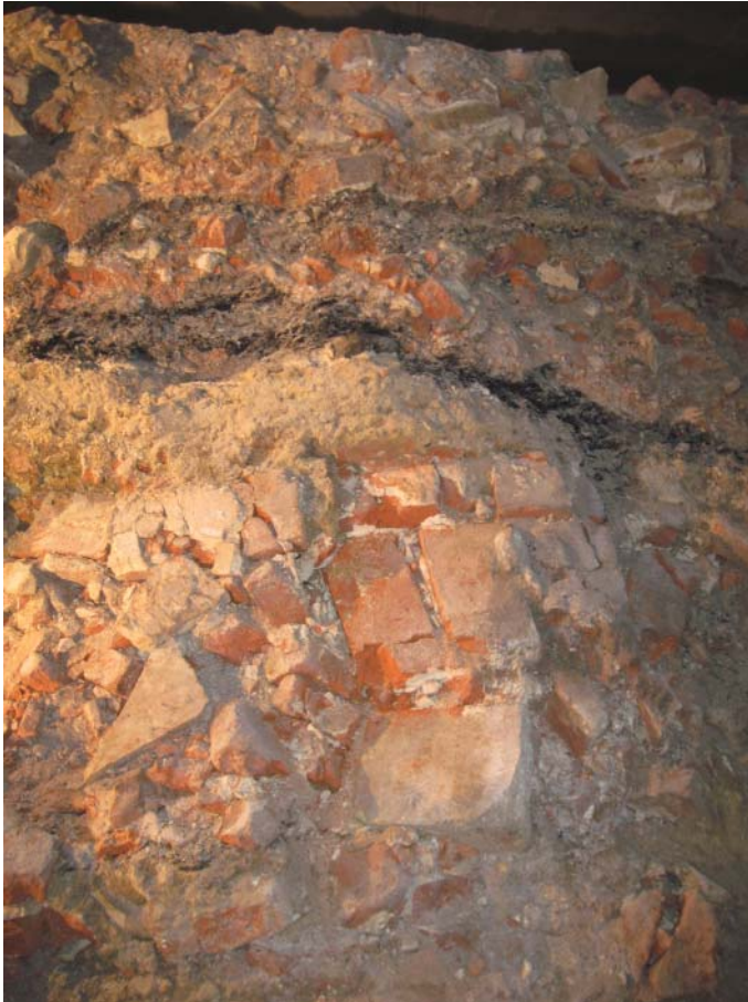
FIGURE 2 Detail of a pile of debris, found in the Aula Magna, left over from the fire of 1731. Consecutive layers of debris can be recognized. The black layer is rich in charcoal fragments from the burnt wood coming from the main banqueting hall at the ground level. Right underneath, the structure of the collapsed vaults from the rooms underlying the main banqueting hall can still be recognized. The bedding mortar of the vaults was sampled (mortar M5).
