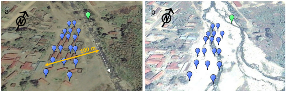
Fig. 15 Zoom of a cluster of destruction in the Nyamwamba valley (location: Fig. 13a). Blue dots are destroyed buildings; green dot is a destroyed bridge. Left pre-flood image GE, March 24, 2006, 0.195°N, 30.02°E. Right post-flood image GE, January 13, 2014, same location. White arrow indicates river flow direction
