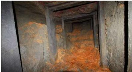
Figure 7: Vertical soil between 2 wooden frames in an unfinished tunnel of the Zonnebeke Dugout (photo Ingenieursbureau Norbert Provoost byba)
