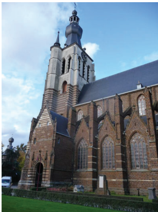
Figure 1. Typical example of the local architecture found along the Demer river: Our Lady's Church of Aarschot. Ferruginous sandstone is alternated with layers of the light-coloured sandy limestone of Gobertange (Brussels Formation).
