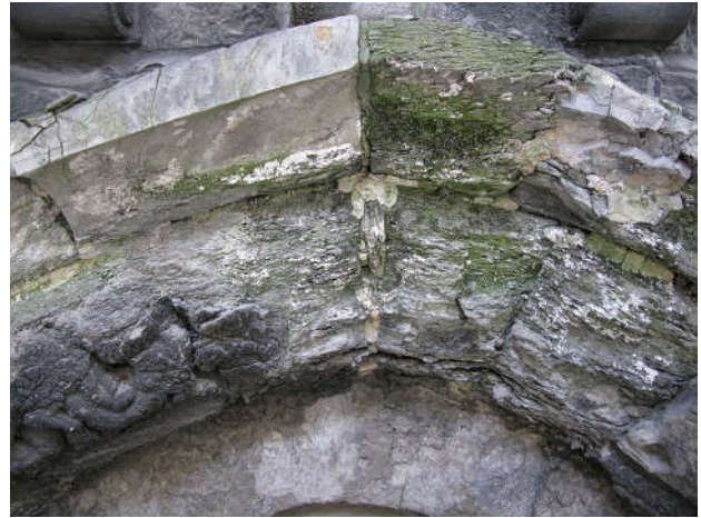
Fig. 5 Summit of the Mantile portal. Black crusts (thick deposits), green algae, mosses and lichens can be identified © KIK-IRPA (Monuments Laboratory)
