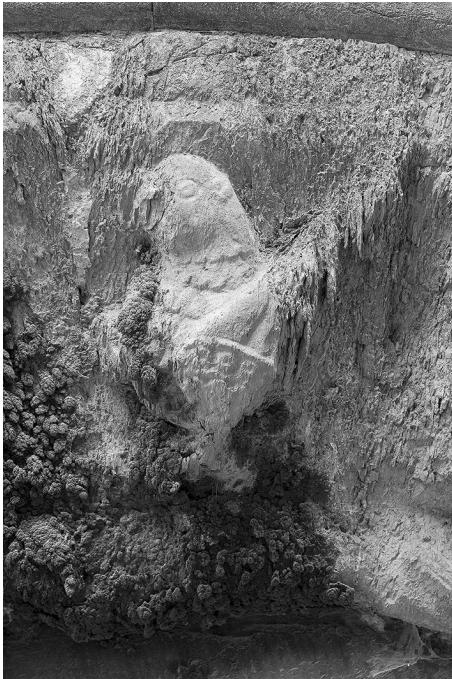
Fig. 3 Edge-bedded block displaying a compact stone core sandwiched by schist-like outer edges (Capitole portal, top of the trefoiled arch) © KIK-IRPA, Brussels
