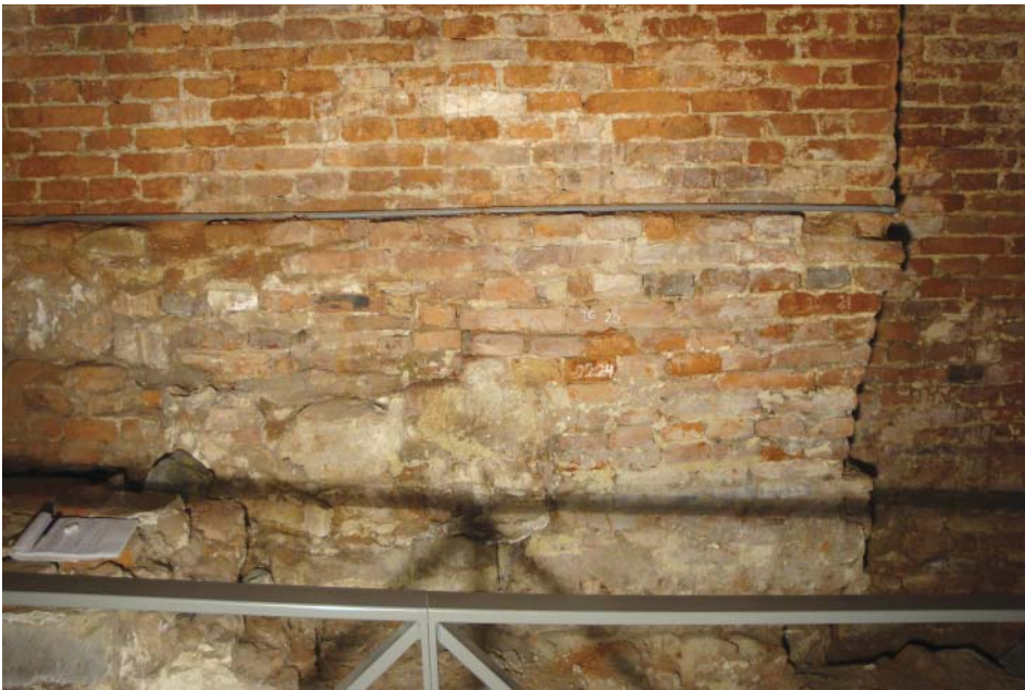
FIGURE 3 Detail of brickwork along Isabella Street.
