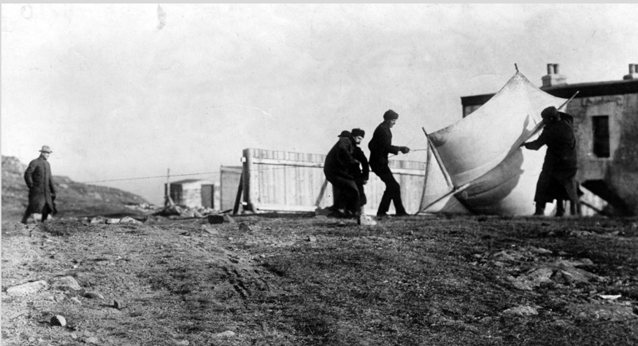
FIG. 2.8 – Guglielmo Marconi and others set up the kite carrying the antenna for the first transatlantic wireless communication, in St. John's, Newfoundland, on December 12, 1901.
