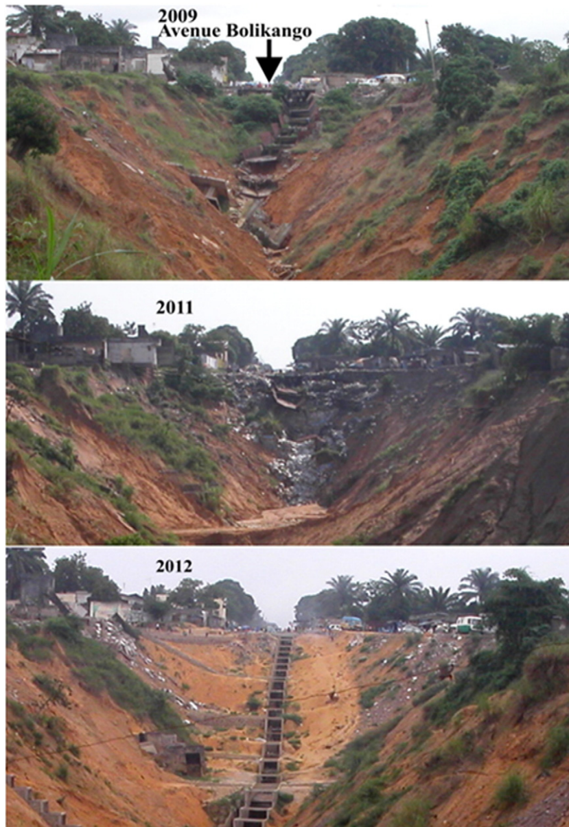
Fig. 7. Mitigation measures at the head of the axial mega-gully of Laloux. In 2009, metallic sheets, intended to protect the gully against further vertical incision and head retreat by runoff from Avenue Bolikango (Laloux Gully, Figs. 1 and 3), were destabilized due to sapping. In 2011, an insufficient amount of sand bags was put in the head to replace the metallic sheets that had partially collapsed. In the foreground the top of a sand dam is visible. This dam caused temporary sedimentation in the mega-gully bottom. In 2012, the metallic sheets were all take away and a huge staircase-like gutter has been constructed.
