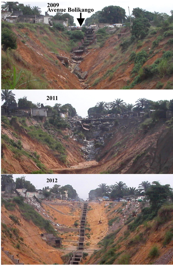
Fig. 6. Axial mega-gully head of Laloux gauche. A construction of metallic sheets, intended to protect the mega-gully head against further vertical incision and head retreat by runoff from Bolikango Street (Laloux gauche, Fig. 1) is destabilized from below. The 2011 picture shows that an insufficient amount of sand bags has been put in the mega-gully head to replace the metallic construction which has partially gone. In the foreground the top of a sand dam, is visible. This dam causes temporary sedimentation in the mega-gully bottom. Finally in 2012 the metallic sheets were all gone and a huge staircase-like gutter has been constructed.
