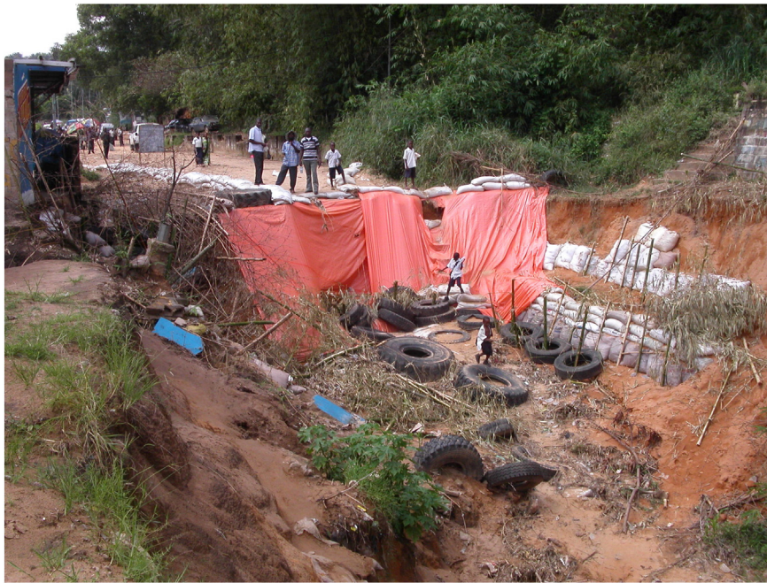
Fig. 5. Tyres, sand bags, canvas, fences of wooden sticks, auto parts and rubbish, to protect the axial mega-gully on the road of Kimwenza, 3 km south of the UNIKIN campus, 2009. The axial mega-gully developed from the plunge pool head of a progressive leak mega-gully behind the back of the photographer. Finally, in 2010, a Chinese contractor has filled up the axial part of the mega-gully and repaired the road. The plunge pool head has been stabilized by a huge massive retaining wall with a concrete gutter to assure a safe outlet of the water in the future.
