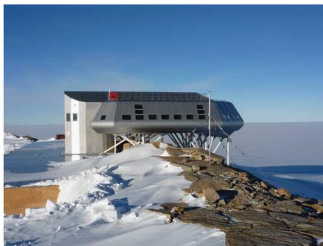
**Fig. 3.** View to the north of the Utsteinen Ridge and the Princess Elisabeth Station. The main wind direction is from the east (right side of the picture). Drifting snow fills the west side (left side of the picture) of the ridge. The main structure is 22 by 22 m and elevates 2–5 m above Utsteinen Ridge.
